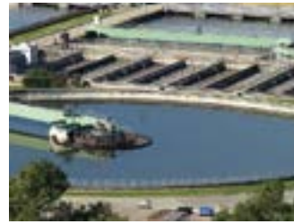
Municipal or industrial wastewater tertiary treatment
